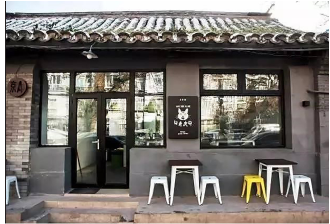
Figure 5: A neighborhood restaurant at Xiang'er Hutong No. 84 before renovation. Photo by MEI Shanshan, published on June 3, 2017 on http://wx.imspender.com/articles/12zhang-hu-tong-zheng-zhi-qian . Accessed on September 16, 2017.
